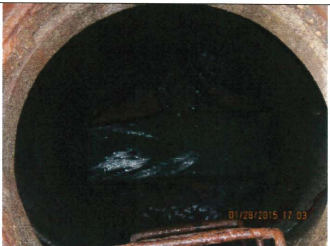
Photo 20: Manhole at Broadway & 2 nd Street
