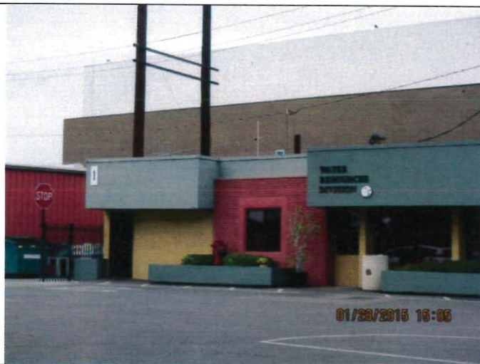
Photo 1: Water Resources Division building
