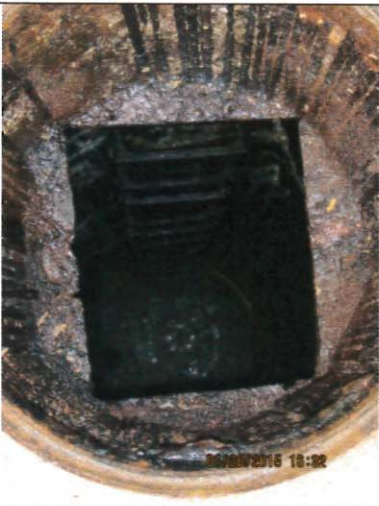
Photo 19: Shutters on the Beach Hotel secondary clarifier
