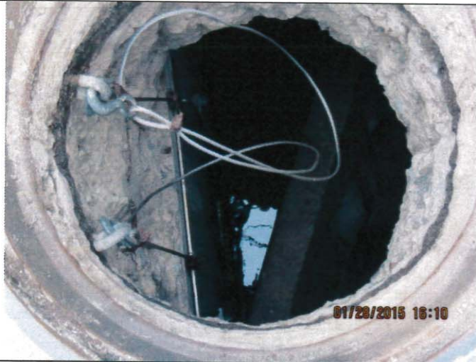
Photo 13: Pico-Kenter low flow diversion system with manually-operated gate (left) and diversion weir (right).
