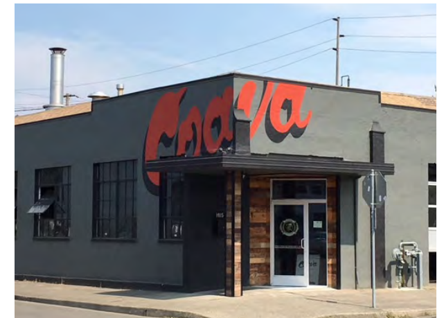
Historically-inspired signs painted directly on building facades
